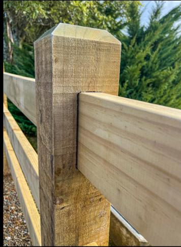
KIWILOCK® Fencing - Interlocking post and rail fencing is an innovative fencing system that is quick and easy to install. The rails are cut to length and slide straight through the machined posts to fit securely with no fixings required.
