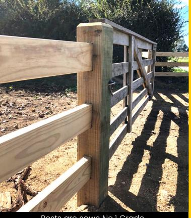
Posts are sawn No.1 Grade Smooth 'dry' rail, Ex 150x50mm No.1 Grade 4.0m Long All posts have bevelled tops Posts are spaced 2m apart
